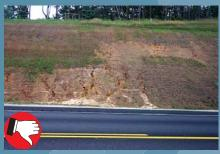
Poor seed establishment on slope. Use seeding in combination with other BMPs (e.g. erosion control blankets) when slopes are steep.
