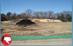
Inadequate ECB to protect this area of exposed soil; additional BMPs are needed. ECB is not trenched or anchored correctly as indicated by sediment at the curb. Spoil piles should also be better protected.
