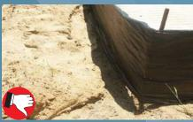
Silt fence is not properly trenched. The lower edge of the fabric must be securely embedded 6 inches in soil.
