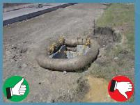
Good application of organic filter tubes to protect the storm drain; however, they are not staked or properly embedded in the soil.
