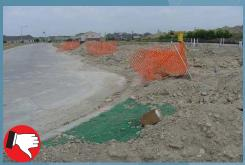
Piles of sediment are inappropriately placed on top of ECBs in the process of digging for utility/water lines.
