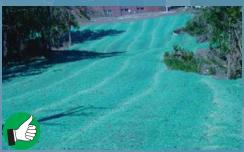
Excellent slope protection. ECBs are correctly installed on this long slope (vertically) and should be installed horizontally on short slopes.
