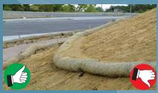
Appropriate use of a series of organic filter tubes to protect a slope; however, accumulated sediment must be removed.
