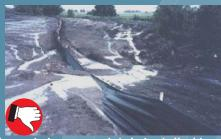
Silt fence is inappropriately installed in an area subject to concentrated flows. A check dam would be more suitable here. There is no wire mesh backing to reinforce the silt fence and wood posts are being used instead of metal.
