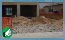
Crushed stone is being used to protect site's exit, allowing for easy access for delivering materials, minimizing tracking, and protecting other BMPs. Note the appropriate placement of sand—on the other side of the BMP.
