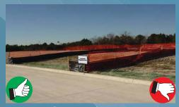
Silt fence, orange fence, and signage are appropriately used to manage concrete waste; however, rock should be placed at the entrance to prevent offsite tracking.
