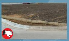
Inadequate organic filter tubes to protect this area of exposed soil; additional BMPs are needed. Tubes need to be re-aligned at the curb and appropriately embedded into the soil.
