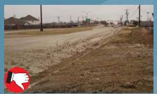
Rock material and geotextile filter cloth are missing. Offsite tracking and sediment loss is occurring. Exit should also be sloped away from the paved surface.
