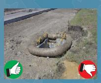
Good application of organic filter tubes to protect the storm drain; however, they are not staked or properly embedded in the soil.
