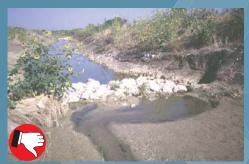
Loose rock check dam is installed incorrectly and erosion of the bank due to flow bypass around the dam has occurred. Check dam must be placed across the entire ditch and partially up the banks.
