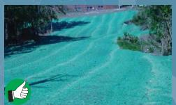
Excellent slope protection. ECBs are correctly installed on this long slope (vertically) and should be installed horizontally on short slopes.
