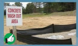
Signage is used properly to identify the concrete washout area.
