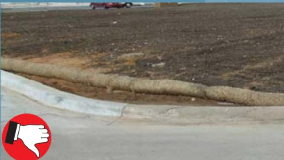
*Inadequate organic filter tubes to protect this area of exposed soil; additional BMPs are needed. Tubes need to be re-aligned at the curb and appropriately embedded into the soil.*
