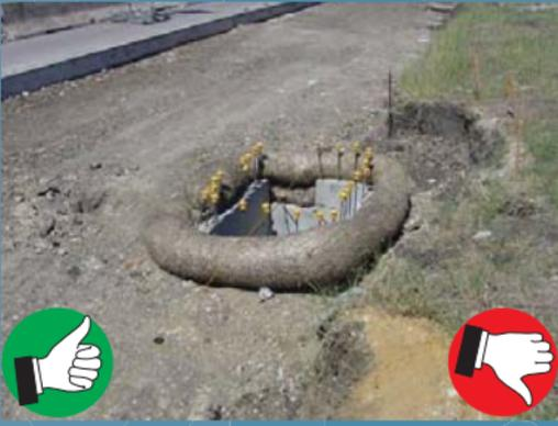
*Good application of organic filter tubes to protect the storm drain; however, they are not staked or properly embedded in the soil.*
