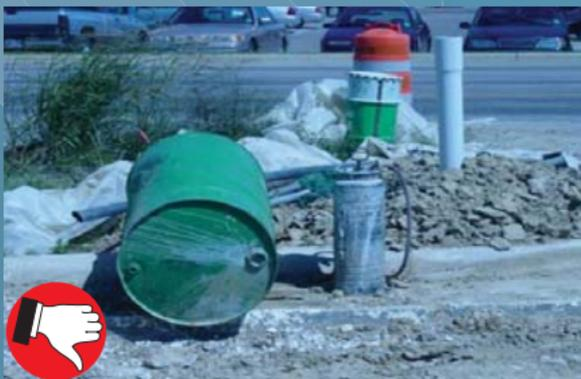
*Chemical storage container is inappropriately discarded, and there is evidence of a spill. Chemicals should be properly stored and disposed of and spills cleaned up immediately.*
