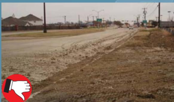
*Rock material and geotextile filter cloth are missing. Offsite tracking and sediment loss is occurring. Exit should also be sloped away from the paved surface.*
