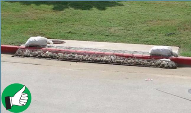
*Excellent use of filter fabric with wire mesh backing and rocks enclosed in wire mesh to protect the storm drain. Protection is secured at top with rock bags to keep in place. Overflow gap allows water from a rain event to enter the storm drain, which prevents flooding of travel lanes.*
