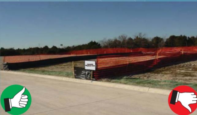
*Silt fence, orange fence, and signage are appropriately used to manage concrete waste; however, rock should be placed at the entrance to prevent offsite tracking.*
