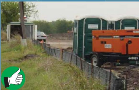
*Portable toilets are placed behind BMPs and away from the street or drainage ways should a spill or leak occur.*
