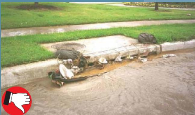
*Poor management of filter fabric and wire mesh to protect the storm drain. Protection is bent and is not flush with the storm drain to properly pond runoff and filter out sediment. Maintenance is not being performed as needed.*
