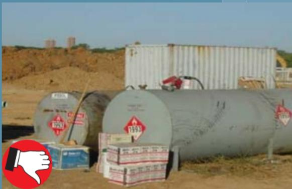
*Inappropriate management of chemicals and other hazardous materials. Gas tanks need secondary containment that is 110 percent of the container. Other chemicals should be stored in an appropriate enclosure to minimize potential of stormwater contamination.*
