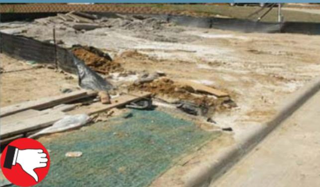
*A washout area has been designated; however, the waste is being managed inappropriately. BMPs surrounding the washout area are damaged and the area is full and concrete should be removed and disposed of properly (recycle where possible). BMPs are absent to protect against offsite tracking and runoff.*
