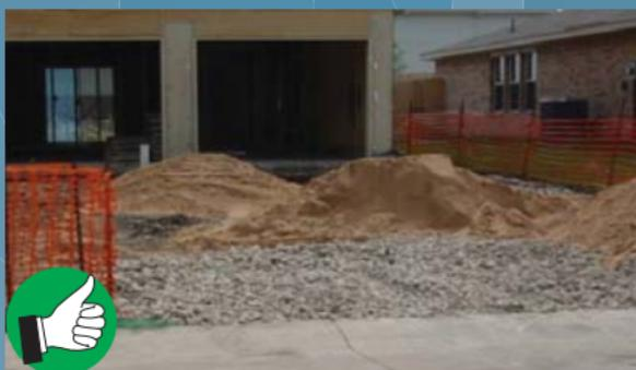
*Crushed stone is being used to protect site's exit, allowing for easy access for delivering materials, minimizing tracking, and protecting other BMPs. Note the appropriate placement of sand—on the other side of the BMP.*
