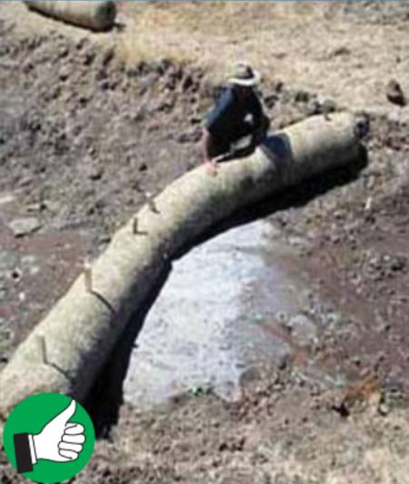
*Check dam consisting of organic filter tube effectively reduces the velocity of this flow as indicated by pooled water.*
