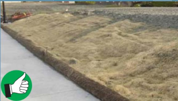
*Organic filter tubes are used with other BMPs to protect an area that may prevent the embedment of other controls.*
