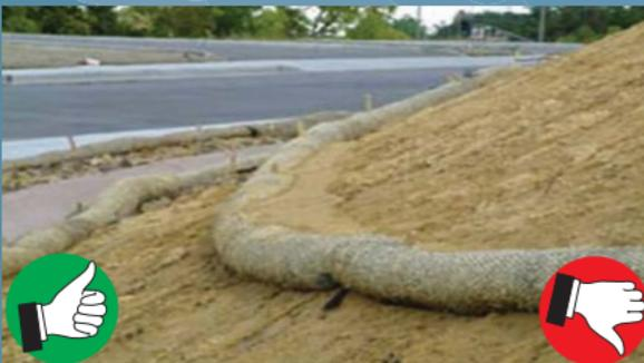
*Appropriate use of a series of organic filter tubes to protect a slope; however, accumulated sediment must be removed.*
