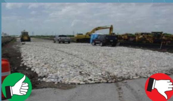
*Good application of stabilized construction exit; however, offsite tracking is still occurring. Voids between stones may be filled with sediment. Fabric and rock should be extended to orange barrel to better transition to paved surface. Good use of barriers to ensure stabilized exit is used.*
